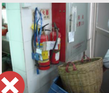
Example of blocking of fire equipment.
