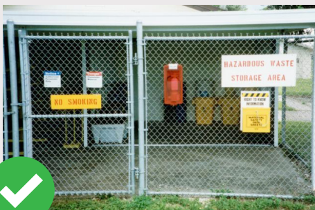
Properly protected hazardous waste storage area.
