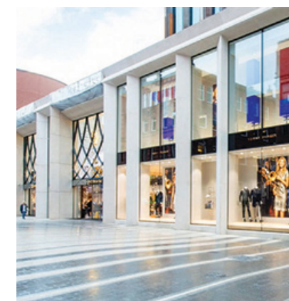
Tommy Hilfiger store in the UK city of Leeds has achieved a BREEAM certification
