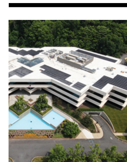
Solar panels on the roof of PVH's offices in Bridgewater, New Jersey
